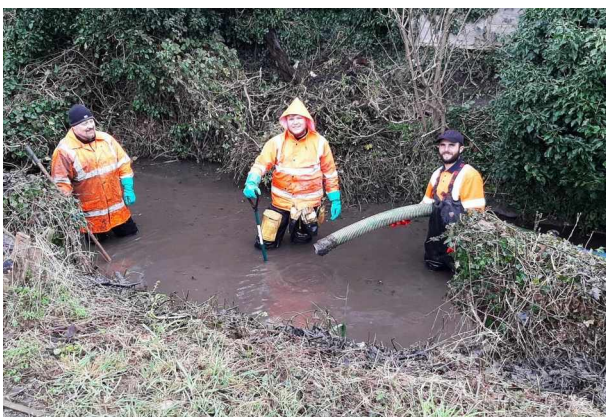
Photos: Pipe used for drawing up the silty water (left); machine that separates silt from water. © Sue Wells
