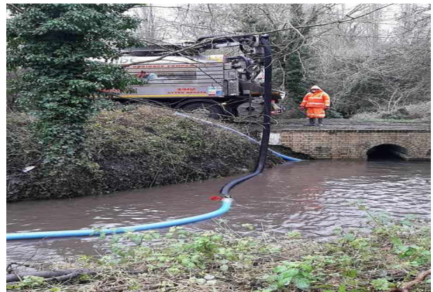
Photos: Pipe used for drawing up the silty water (left); machine that separates silt from water. © Sue Wells
